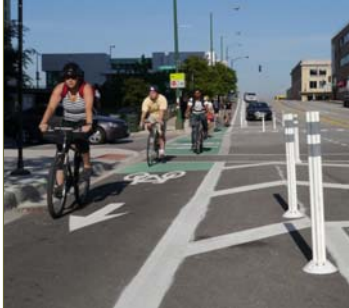
Buffered Bike Lane (with delineators)
